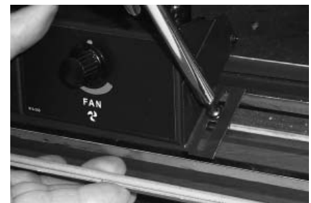
Secure right side with one screw.
