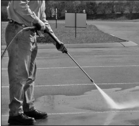
Figure 12 - Optimum angle to cleaning surface
