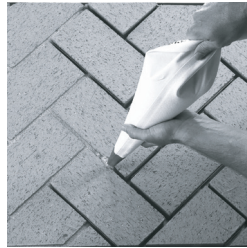
Figure 16 - Grouting Brick
