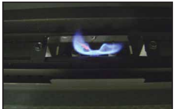
Figure 3.1 IPI Pilot Flame Pattern
