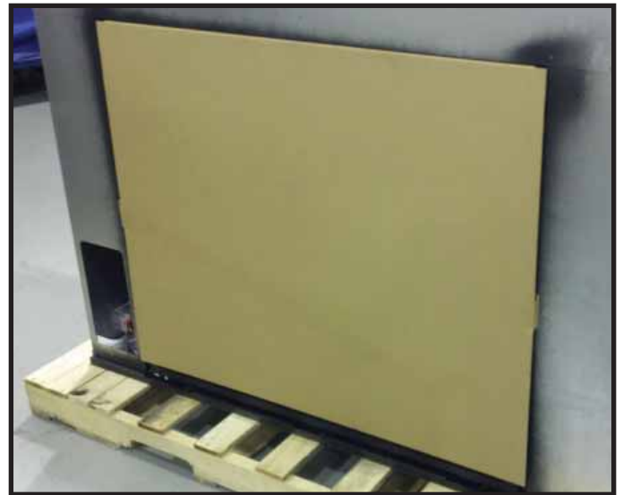
Figure 13.6. Splatter Guard Installation
