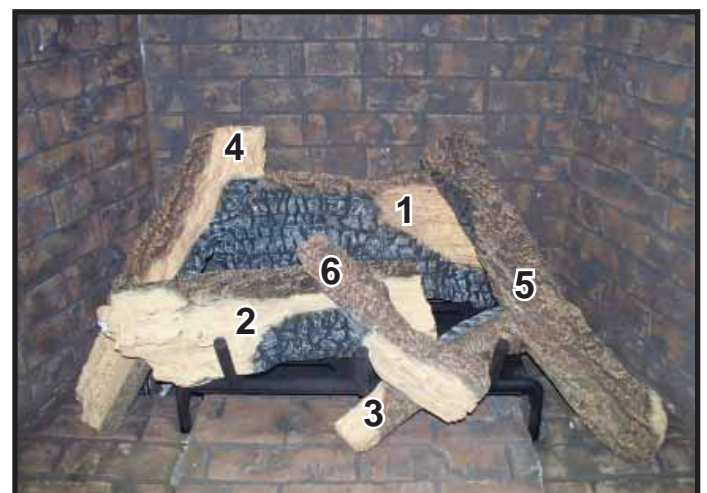
Figure 14. Log Set Installed.
