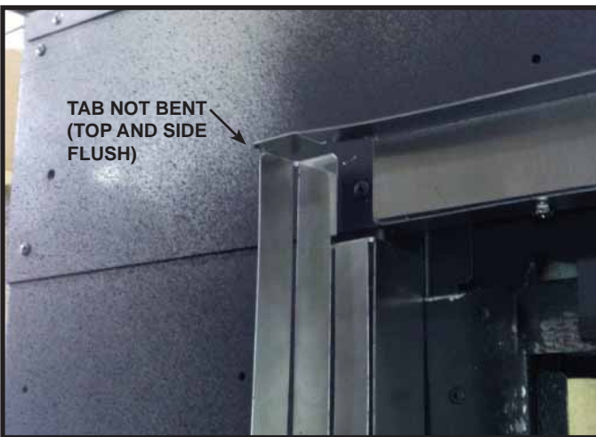
Figure 13.5 Finishing Template Bend - Operable Doors
