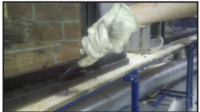
Figure 14.5 Inserting Glass Clip Tool
