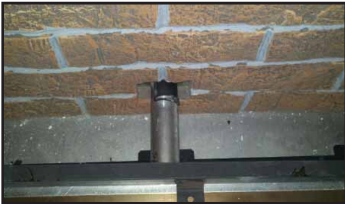
Figure 14.11 Air Shutter
