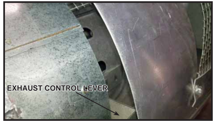
Figure 7.10 PVK-80 Control Lever Adjustment - Open
